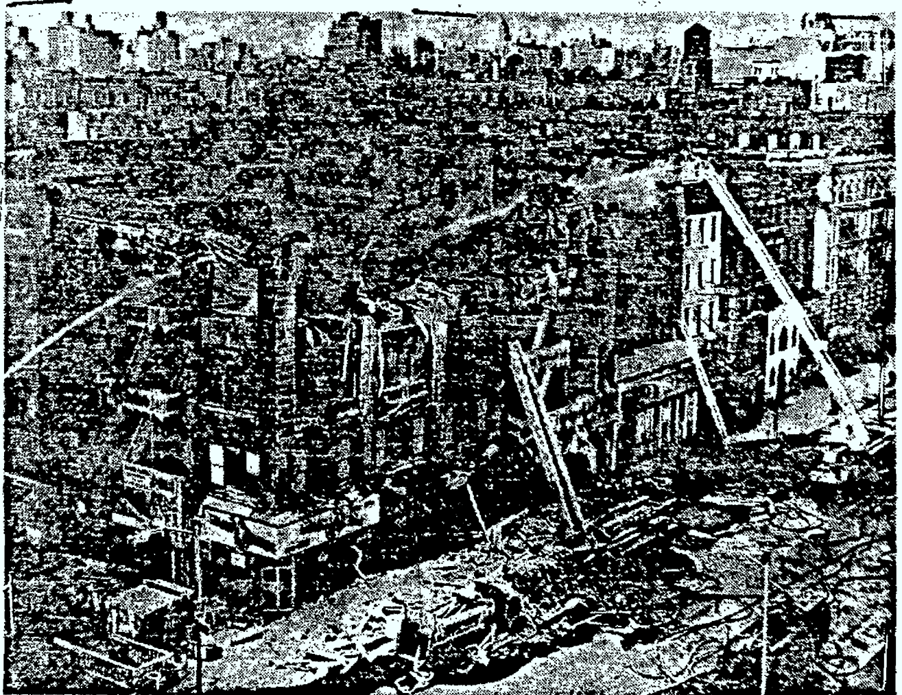
AVALANCHE OF BRICKS partly buried this fire truck and engine on 116th St. and Lenox Ave. after roof collapsed and a brick wall crashed into the street following an explosion and fire that destroyed Black Muslim Mosque at 102 W. 116th St. early yesterday morning. Fire truck at right pumps water into the smoking debris. Herald Tribune—UPI
